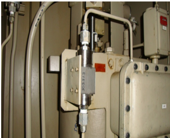
Fig15: New 96FG Installed
