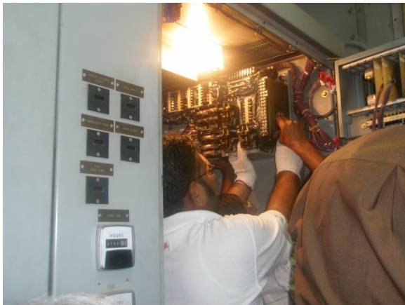
Fig3: Black Start Inverter Installation
